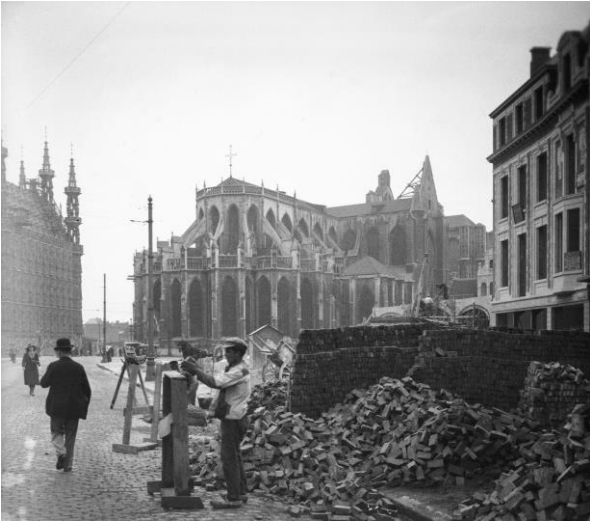
Figure 7: Georges Monnoyer de Galland/Gustaaf Verriest. Leuven, c.1920. Brickies assemble recuperated stones intended for reconstruction works on the Brouwershuis by the recently laid out Maarschalk Fochplein. Stadsarchief Leuven.
